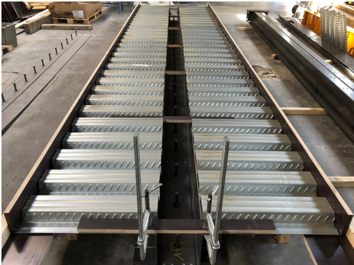
(a) Positioning of the steel decks
