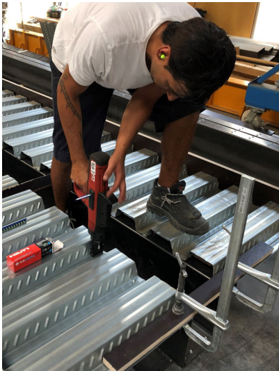
(b) Nailing of the steel decks
