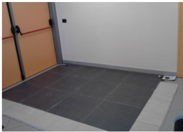
(a) The installed floor prototype
