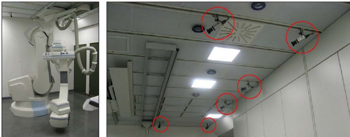
Figure 3.6: Left) Zeego robot from Siemens. Right) Picture from the intervention room at Klinikum Grosshadern, Munich, where the multi-camera system is installed.
