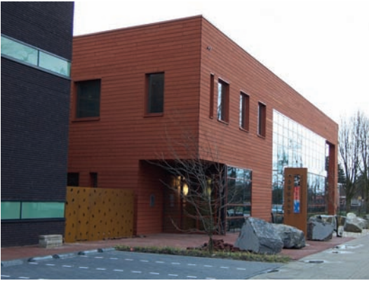
Open Cladding: Plato®Wood Norway spruce with Olympic Stain Location: Helmond
