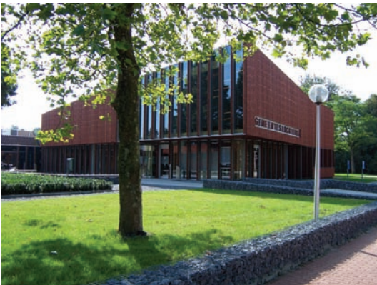
Open cladding: Plato® Wood Norway spruce Location: City hall of Slochteren
