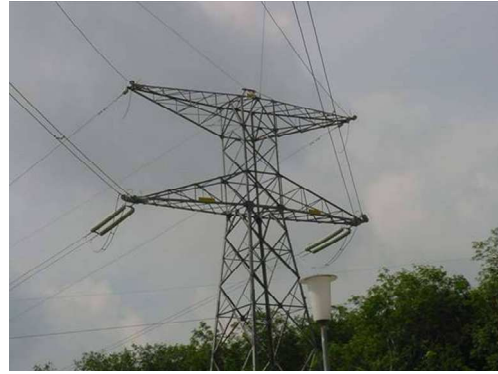
b) 300 kV, 300 MW DC Transmission line
