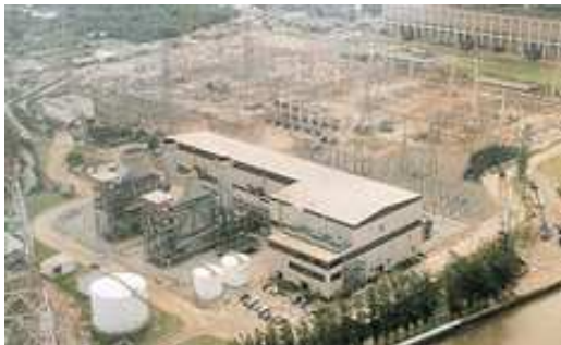
c) 2288 MW, South Bangkok Power Plant, Samut Prakan province
