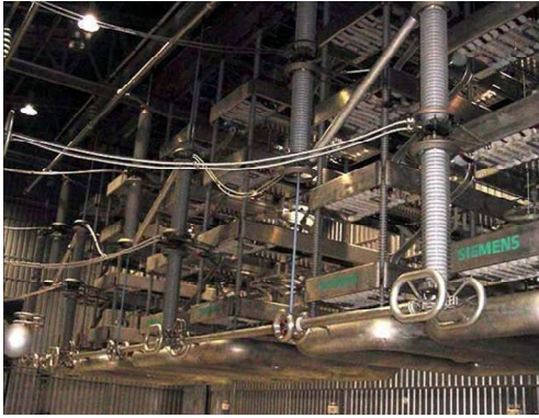
a) Thyristor converter valves
