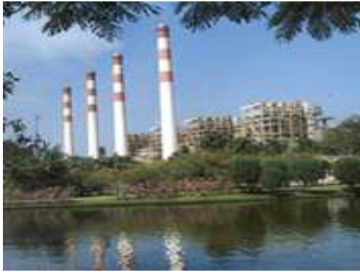
a) 3680 MW, Bang Prakong Power Plant, Chachoengsao province
