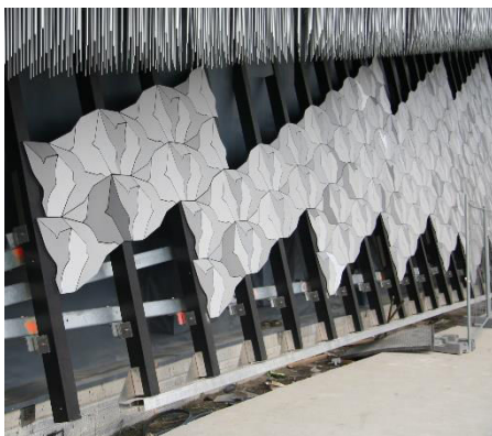
Figure 50. Laser-cut aluminum façade tessellation for the Paris Philharmonic, by Jean Nouvel. 2014. Photo O.GÁMEZ
