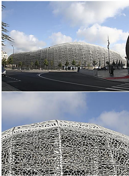
Figure 61. Façade panels derived from a digitally-made biologic-like pattern. Two types of pattern are repeated and adapted over a manifold set of panels whose dimensions change in function of the stadium's geometry. Paris Rugby Stadium at Boulogne-Billancourt, by Rudy Ricciotti. 2007. Photo O.GAMEZ
