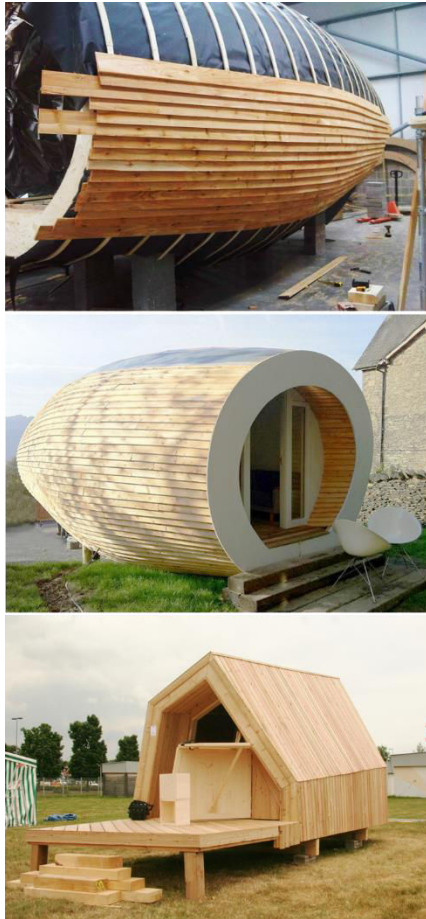
Figure 144. Top. English cedar siding is curved following the pod's geometry. Middle. The Glam Pod in its finished state. On gaukrogerandpartners.com Bottom. Cabin (tiny house) designed and built by students at the wood challenges ( Défis du bois ). Photo O.G
