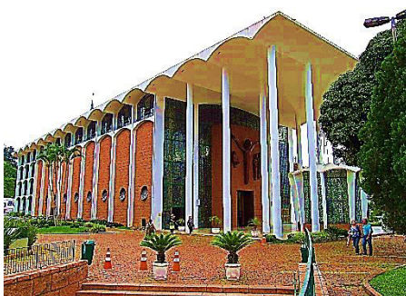
Figure 18. Vermillion granite façade at the Blumenau Cathedral by Gottfried Boehm. 1958, Photo O.GÁMEZ
