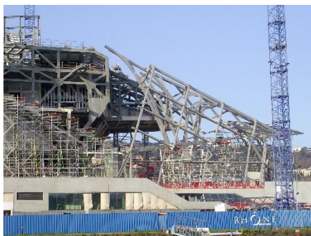
Figure 36. Bearing and façade structures for the Confluences Museum at Lyon-France, by Coop Himmelblau. Photo 2012, O. GAMEZ.
