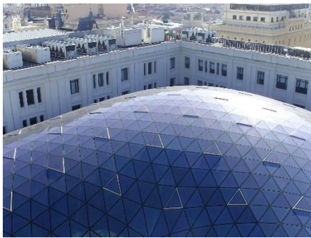
Figure 43. Blob glazed-roof for the Communications Palace, by Arquimedia, Madrid 2011. Photo, O.GÁMEZ
