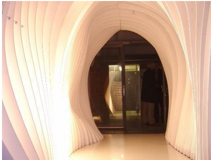
Figure 142. Layered timber structural prototype at “Les Grands Ateliers”, Lyon-France, 2012. Photo O.G
