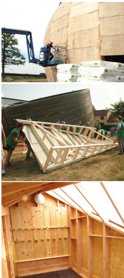
Figure 139. Top. Plywood used as structural material for the Solar Energy House project (see section 5.5). Middle. Moisture-resistant particle board used as roof sheathing at the wood challenges 2015. Bottom. OSB panels used as wall sheathing at the wood challenges 2016. Photos O.G.
