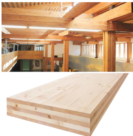
Figure 138. Top . Glulam beams. Vincent Van Gogh High School by Cartignies-Canonica architects, 2006, Blénod-lès-Pont-à-Mousson – France. Bottom . A CLT panel.
