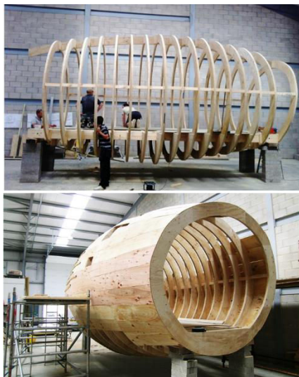
Figure 143. Top. Glam Pod's timber framing seamlessly decreases diameter towards the extremities creating a varying frame-sizing. Bottom. Plank-based sheathing system discontinuously follows the structure's curvature. On: gaukrogerandpartners.com 146
