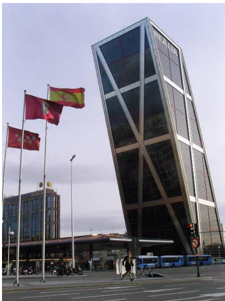
Figure 31. Skewed geometry of the Kio Towers by Phillip Johnson, 1989-1996. Photo O.GÁMEZ.
