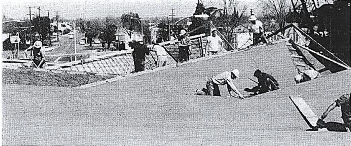
PEAKED ROOF. Workmen put the finishing touches on the Yuba City, Calif., Bank's peaked roof, the first application of ChemComp expansive cement
