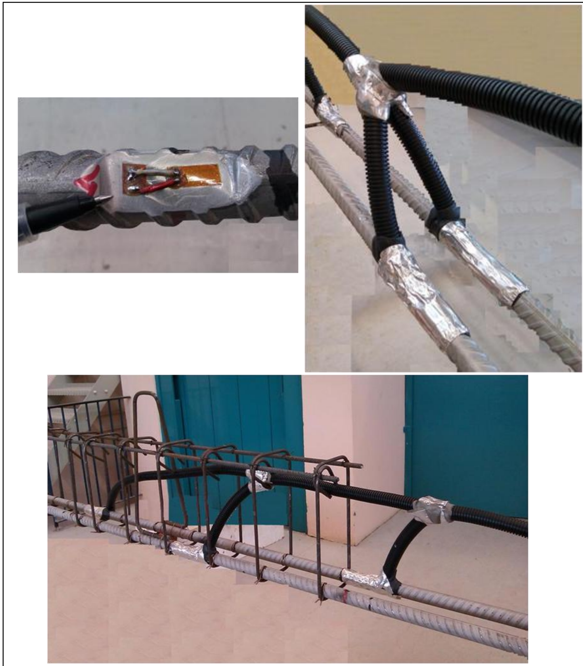
Fig. 3.17. Strain gauges on the reinforcing bars
