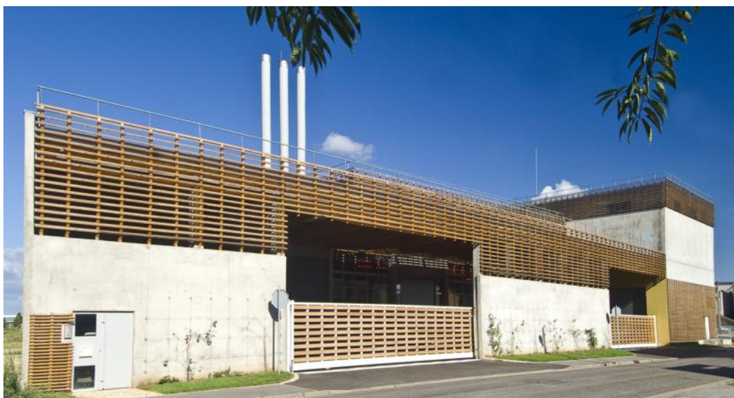
Figure 5 - Chaufferie biomasse Victor
